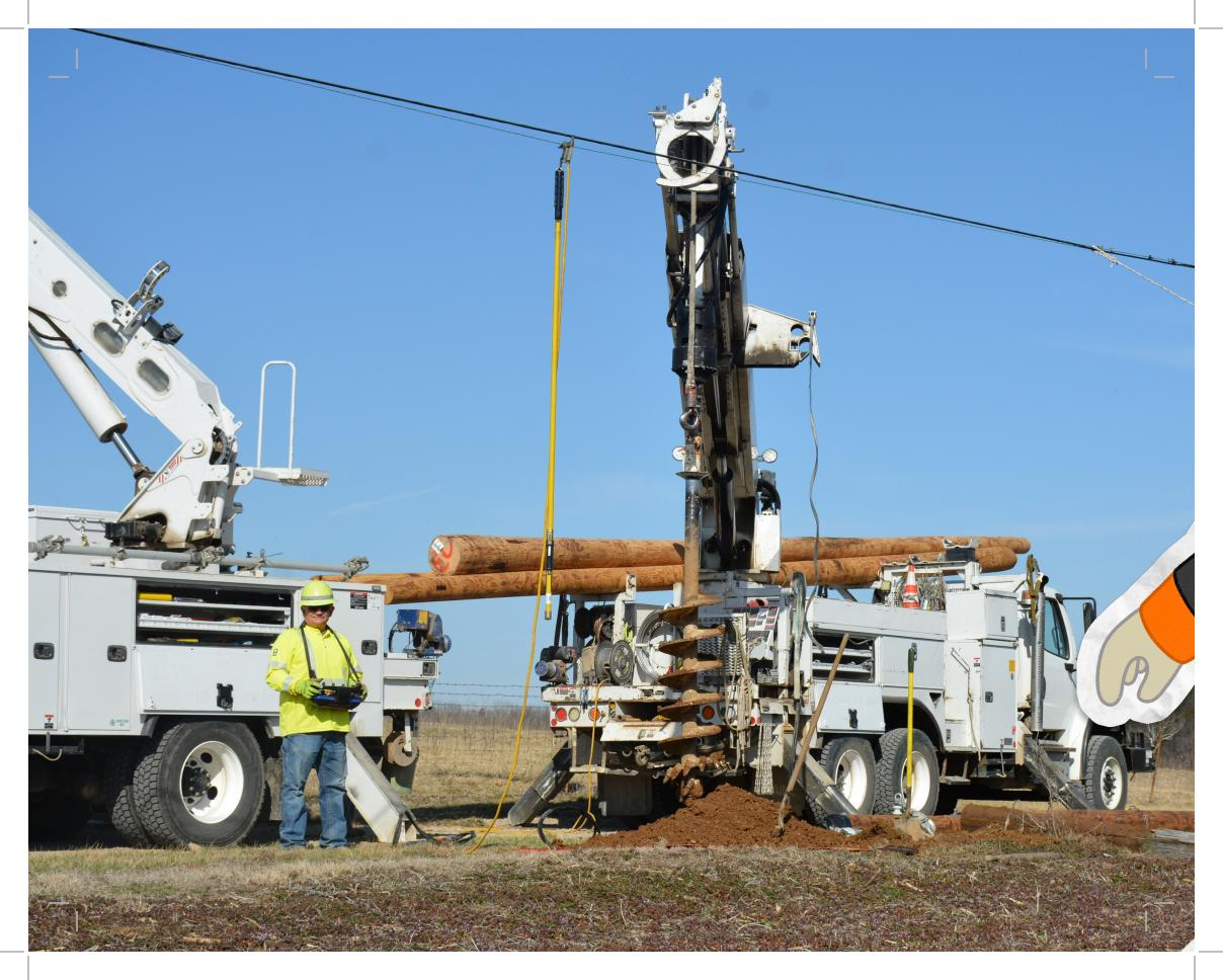
To make sure the hole is big enough for a new power line pole, we use a big drill on one of our trucks called an auger. You can see Danny working the remote controls to make the auger drill down and make the hole!
