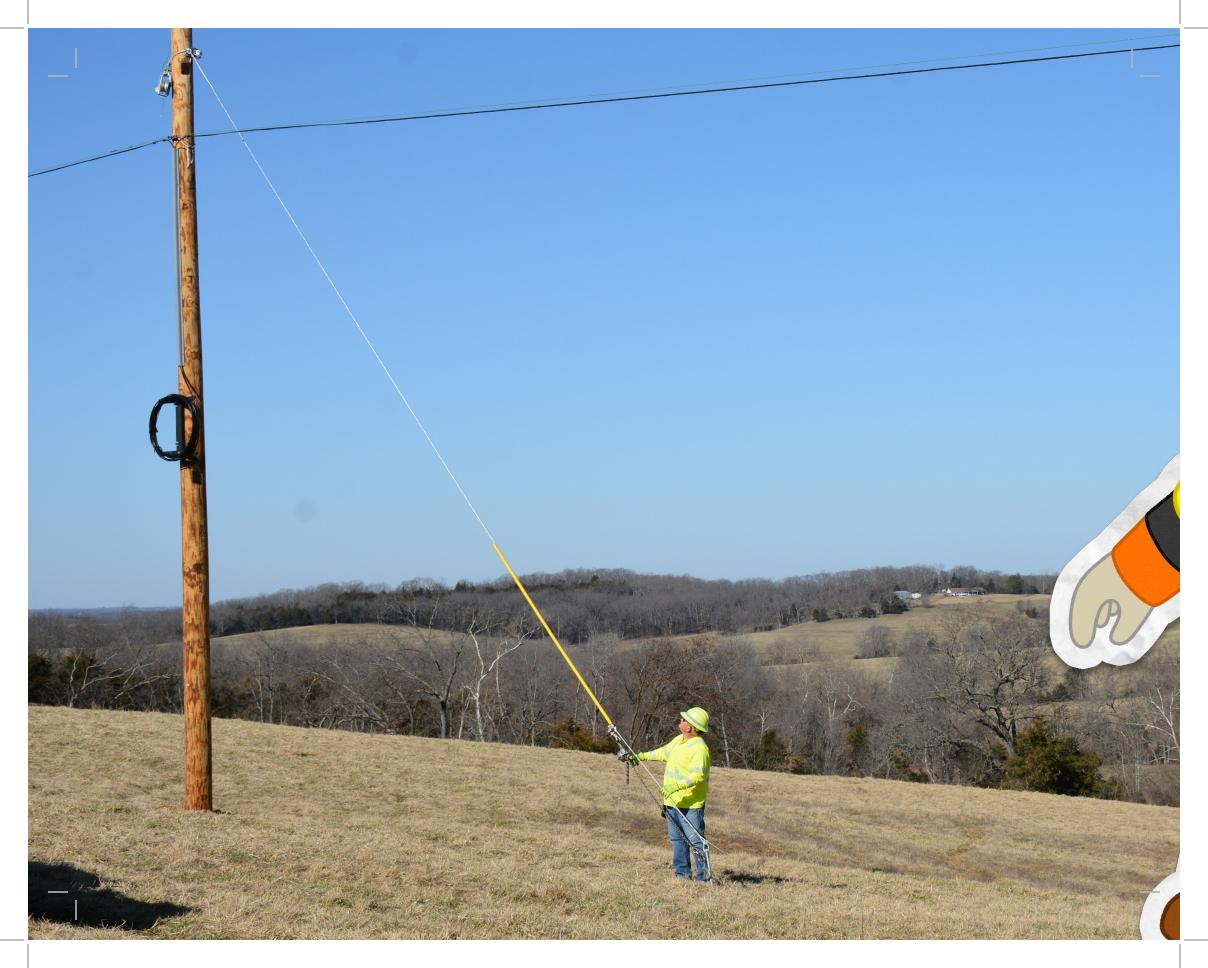
Once the hole is filled, we add a guy wire from the pole to the ground. This helps to support the pole especially in areas with strong winds!
